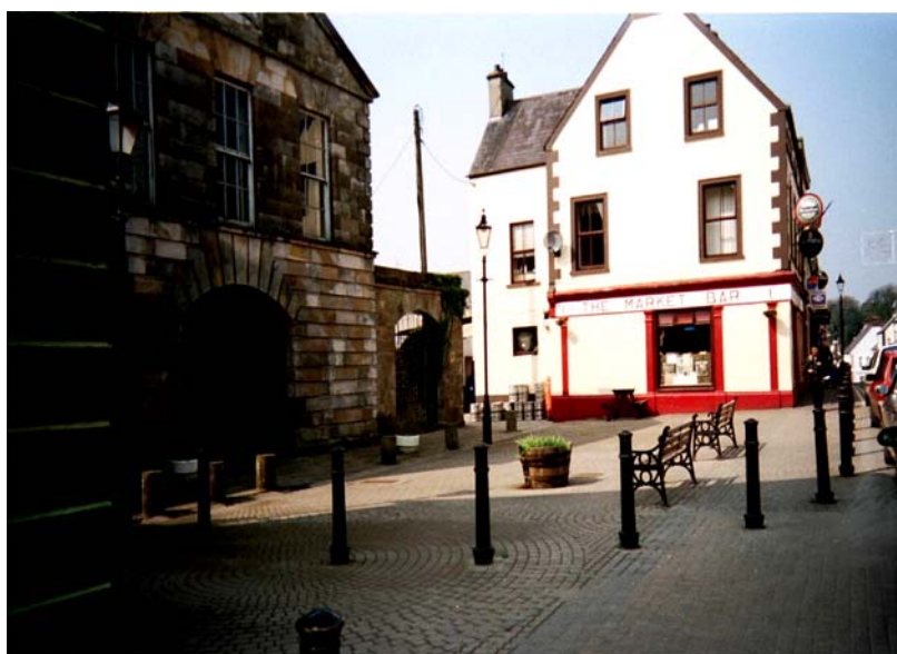
Photo 7.8: Public square in Manorhamilton. Additional planting and street furniture would improve the square. A use for the building on the left of the square should be found.
