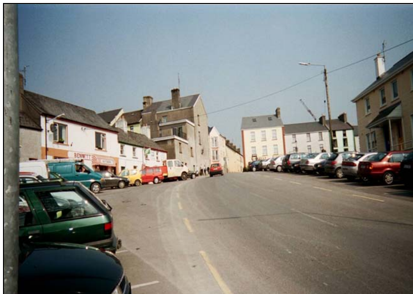
Photo 7.7: Approach to Manorhamilton from Carrick-on-Shannon. The former Burger Magic building (centre left) is highly prominent, as is the on-street car parking.
