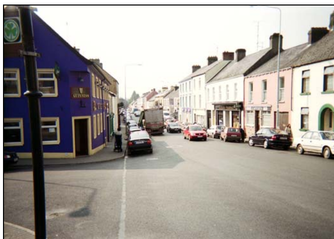
Photo 7.3: Main Street, Ballinamore. The buildings are generally considered in good condition and the overall streetscape is attractive, though on the dominance of on-street car parking is of some concern.
