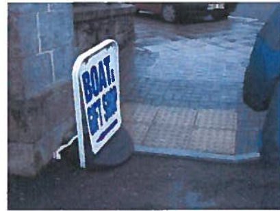
Example 14 ~ Sandwich boards Obstructing tactile pavement markers
