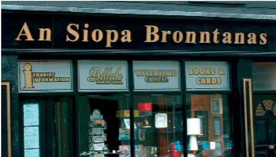
The existence of an over-deep fascia area can completely spoil shopfront proportion. Overall fascia panels should be provided as an integral part of the shopfront, and should be of a depth appropriate to the size of the building and the proportion and the length of the shopfront. The construction of fascias extending above the level of first-floor window sills, and the obscuring and defacing of windows or other architectural details, such as string courses, friezes, cornices, is unacceptable.
